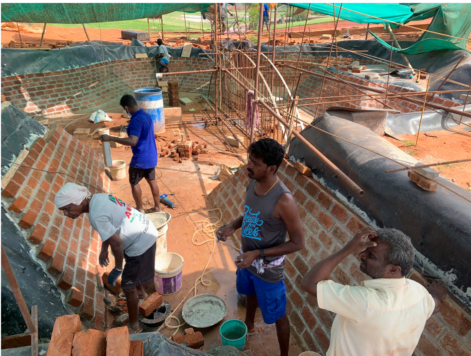
Masons work in the Garden of Utility
